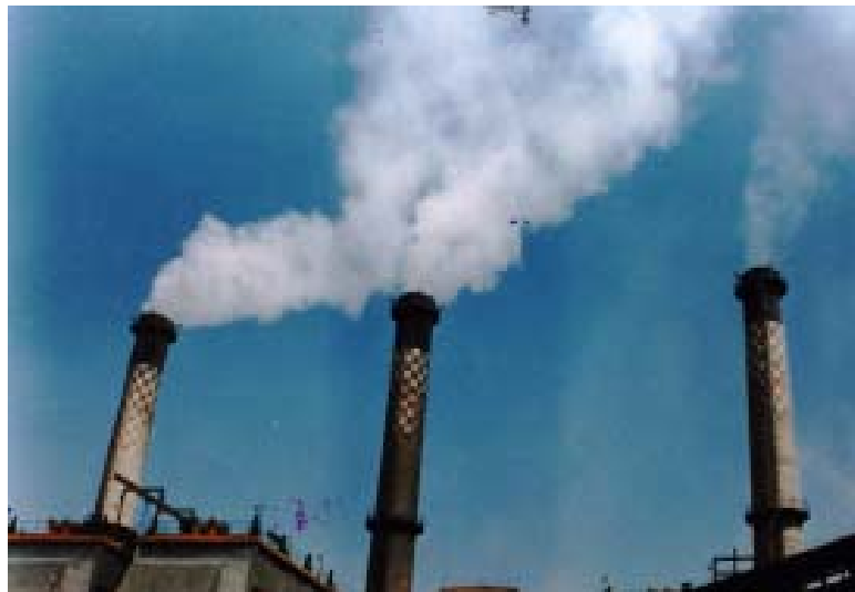
Stack#2 (first from right) is with ammonia conditioning at Punjab State Electricity Board (PSEB) Plant, Bhatinda, Punjab
