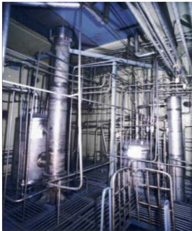
Uranium Thorium Separation Facility
