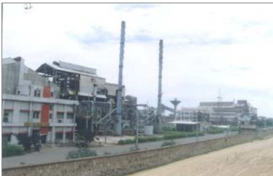
A view of Synthetic Rutile Plant and Mineral Separation Plant at OSCOM
