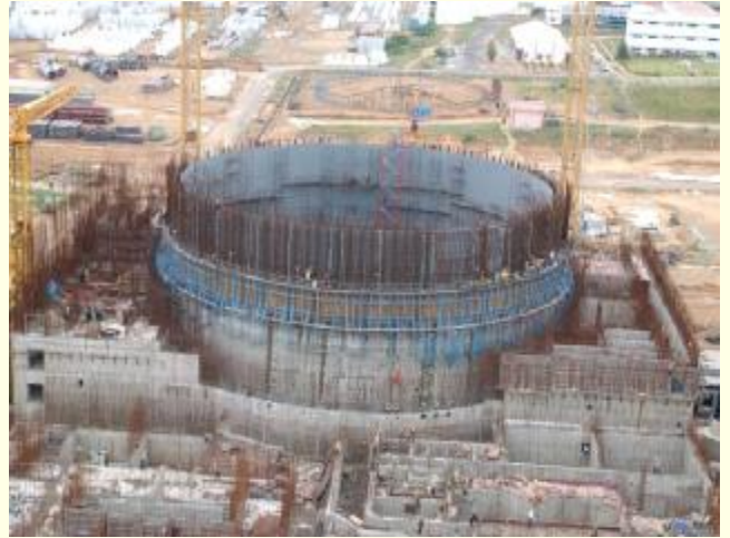
Reactor Building of Kudankulam Unit-2
