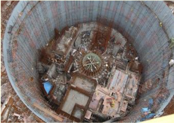
Reactor Building of Kudankulam Unit-1
