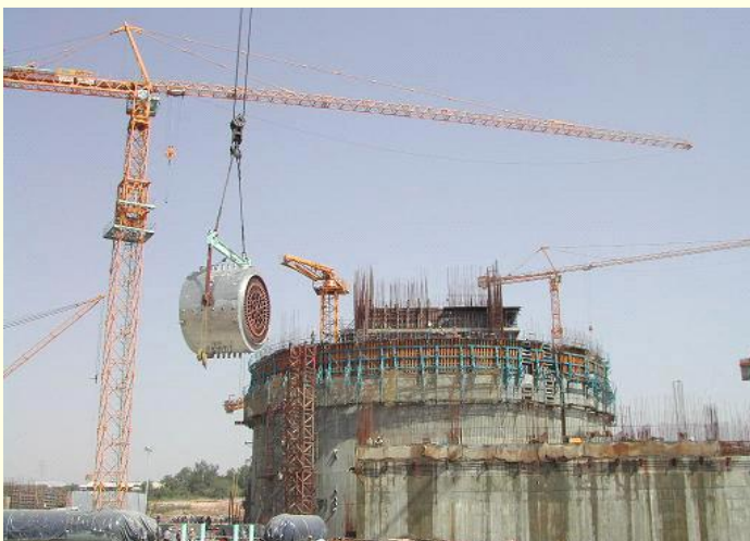
Reactor Building of Rajasthan Atomic Power Project Unit-5
