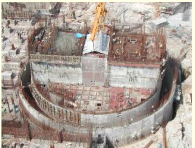
Reactor Building of Rajasthan Atomic Power Project Unit-6
