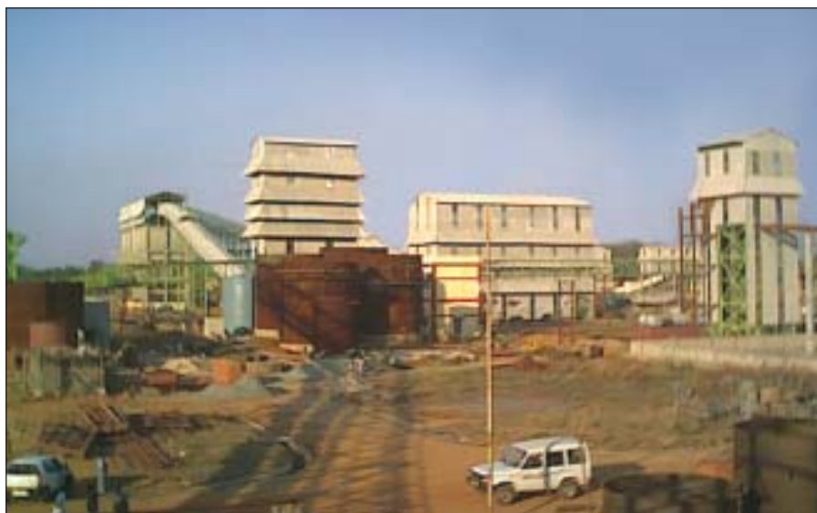
Uranium Processing Plant under construction at Turamdih, Jharkhand
