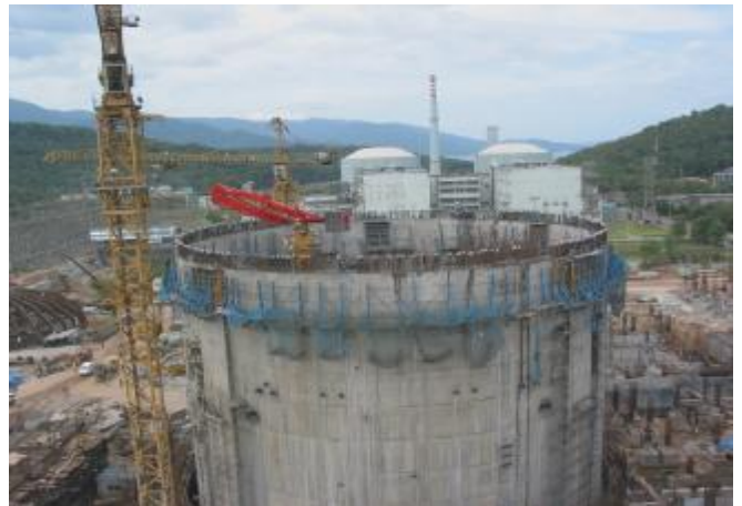
Reactor Building of Kaiga Atomic Power Project-3&4
