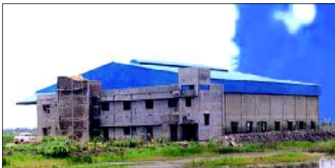
Radiation Plant setup at Kolkata by M/s Organic Green Foods
