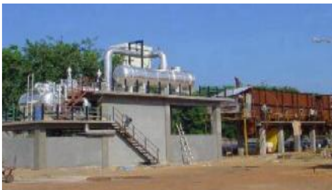
4500 m 3 /day Multi-Stage Flash (MSF) Plant under construction at Kalpakkam
