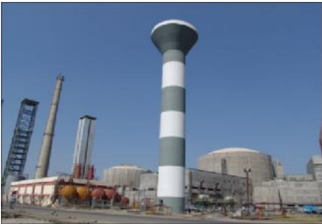
Tarapur Atomic Power Project-3&4
