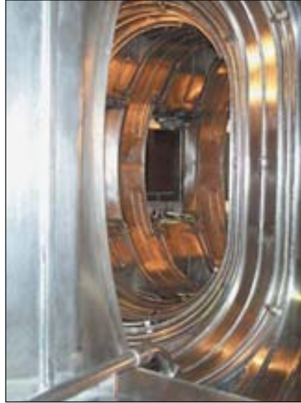
Figure 9: A view of vacuum vessel
