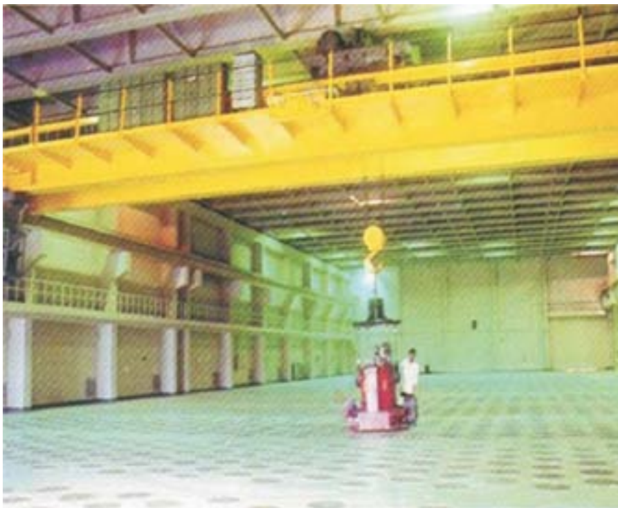
Interim Storage facility for Vitrified Waste at SSSF, Tarapur
