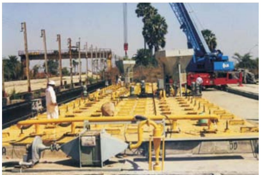
In-situ solidification in Reinforced Concrete Trenches
