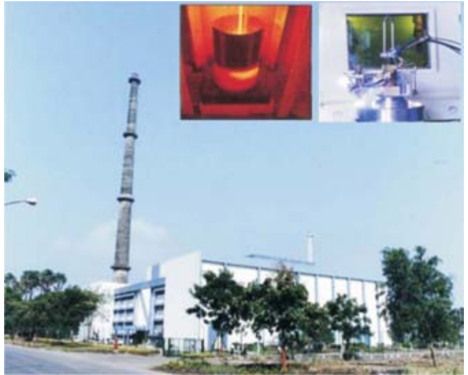
Waste Immobilisation Plant, Trombay. Inset showing pouring & welding of vitrified waste product canister
