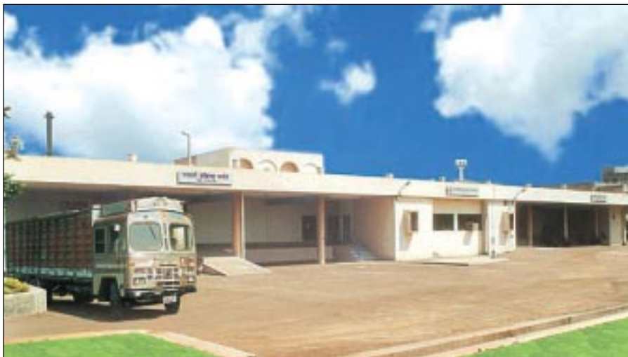
Radiation Processing Plant at Vashi, Navi Mumbai
