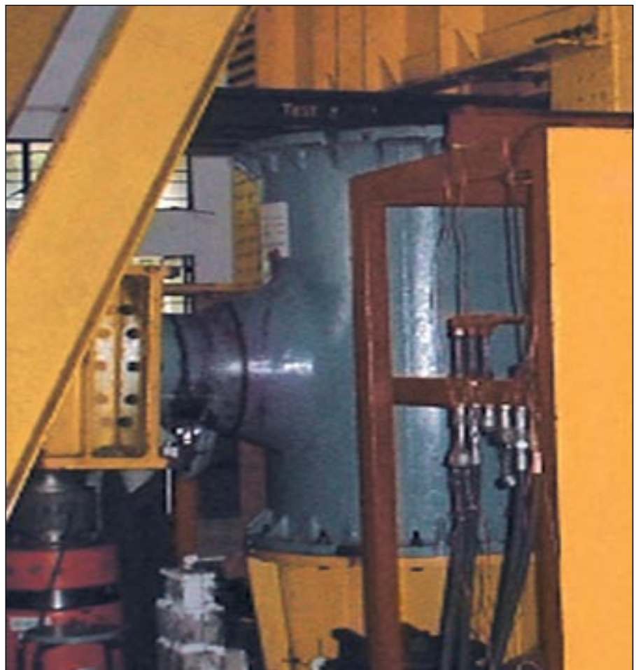
Leak-Before-Break tests of 500 MWe FBR Steam Generator Shell Nozzle Junction at the Structural Engineering Research Centre, Chennai, Tamil Nadu.
