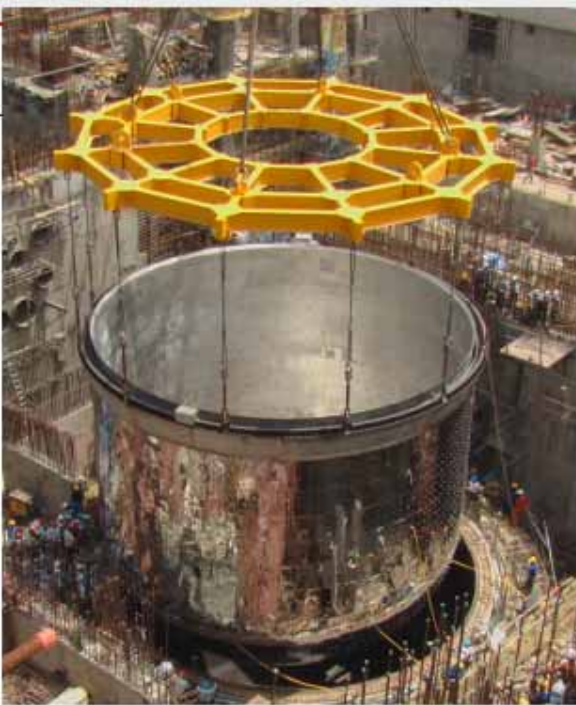
Construction site with Safety Vessel under erection
